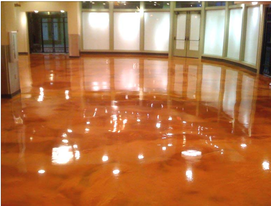
Henry Ford Hospital in Michigan chooses REFLECTOR™ Enhancer Flooring System over tile, wood and even inexpensive VCT.
